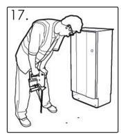
Drill four holes using a 16mm masonary drill to a minimum depth of 80mm. Remove concrete dust from holes with an air blower/brush.
